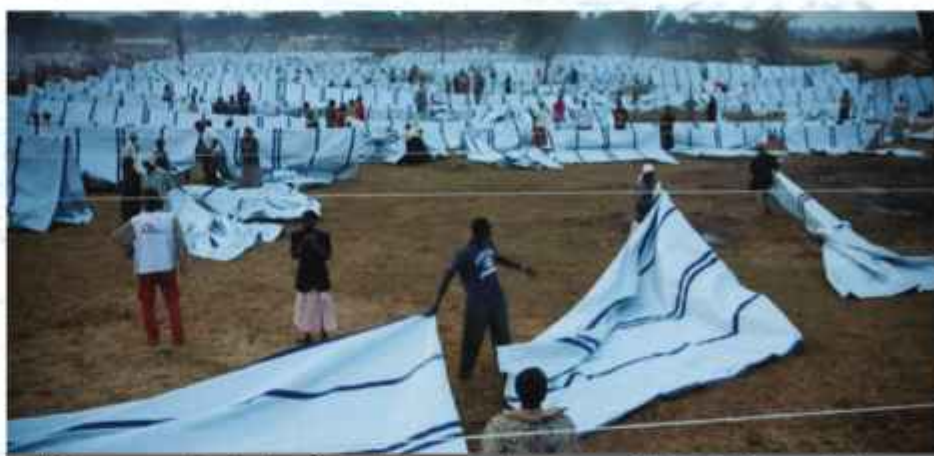
MSF teams suspend rectangles of tarpaulin from ropes strung across a field to make thousands of emergency shelters in Endebess, Kenya, for people whose houses burned down in electoral violence in December 2007. Photograph © Brendan Bannon
