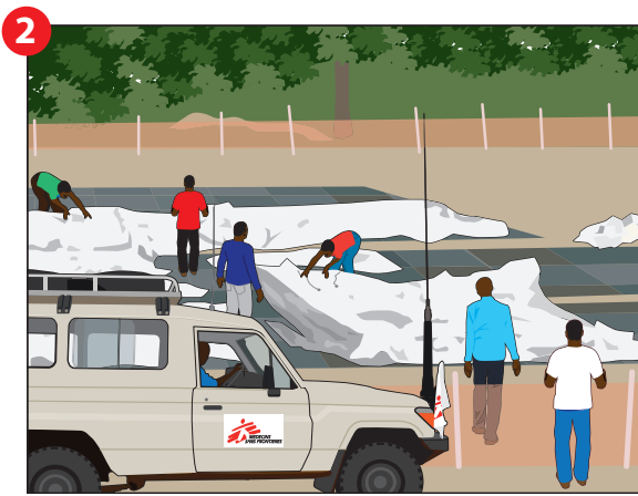
2 The tents are inflated by mechanical air pumps, with each tent equipped with pressure gauges to adapt to changing temperatures. Teams working 24 hours a day can have the full nine-tent structure erected in three days.
