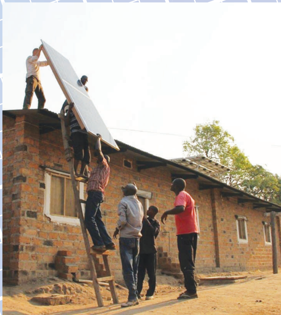
Team members lift a solar panel onto the roof of Shamwana hospital to provide electricity for the off-grid hospital. The solar solution will replace approximately 1,000 litres of diesel per month.
